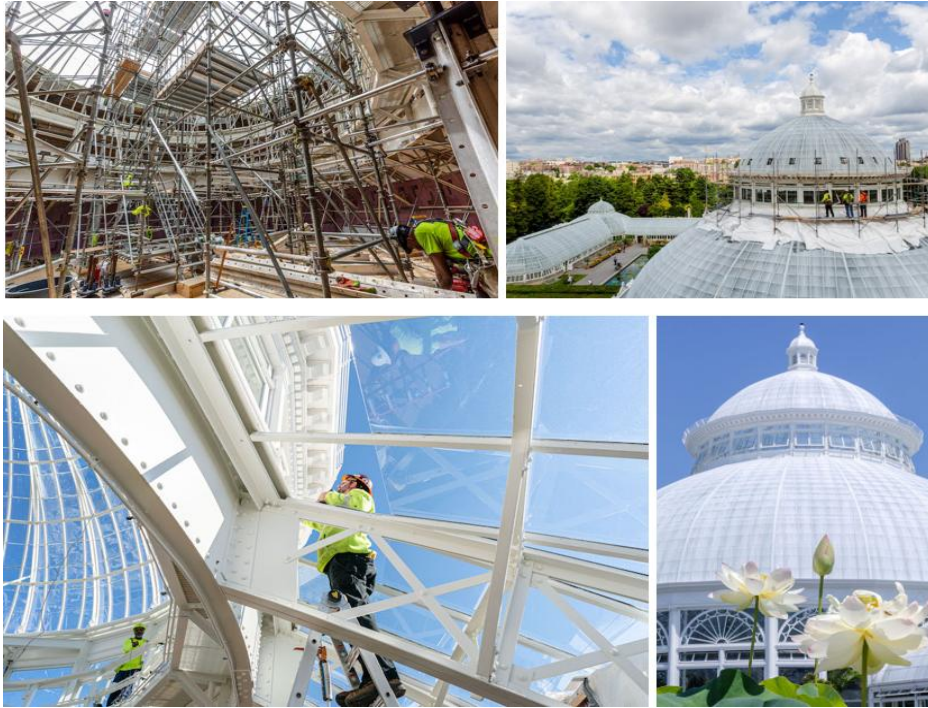
Figure 10. Restoration work of a Victorian greenhouse ( https://www.bdcnetwork.com/famed-dome-historic-glasshouse-revived-its-rightful-glory )
